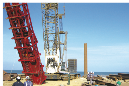
秘鲁D128柴油锤 Project in Peru. With D128
