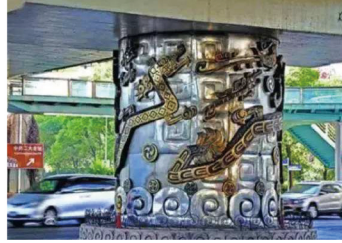
上海延安路高架项目 Yan'an Elevated Expressway, Shanghai
